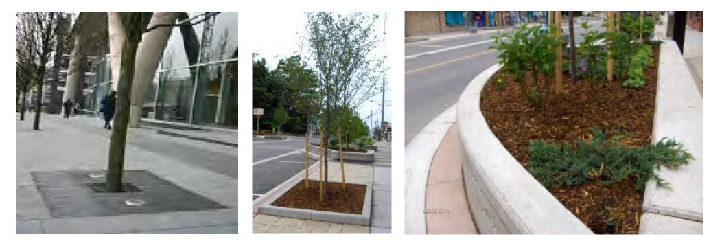
Figure 24, 25 & 26: Precedent Imagery Of Tree Grate, Planting Bed Curb And Seat Wall Treatments
