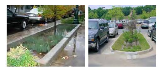
Figure 206 & 207: Rain gardens and bioswale parking areas is an example of the low impact development (LID) approach to storm water management.
